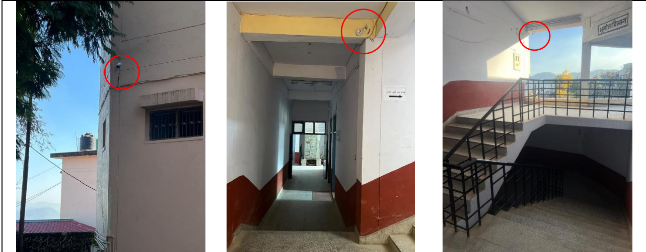
Various CCTV Cameras installed in the college premises for safety and security purpose
